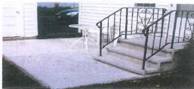
Precast Step on Brick Patio
